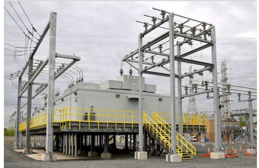
New Equipment Raised Above Flood Elevations
