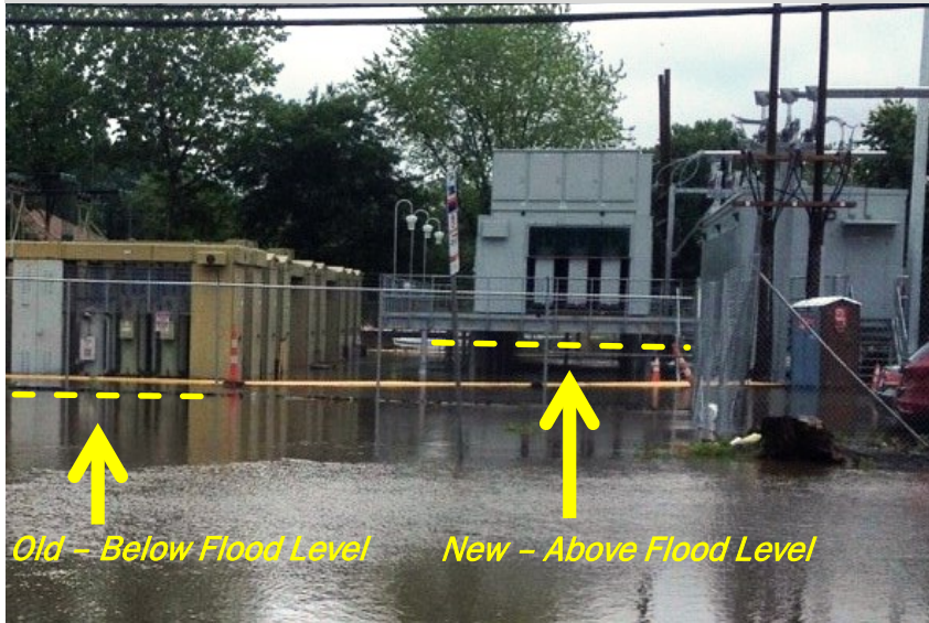
Old Station Below/New Station Raised Above Flood Elevations
